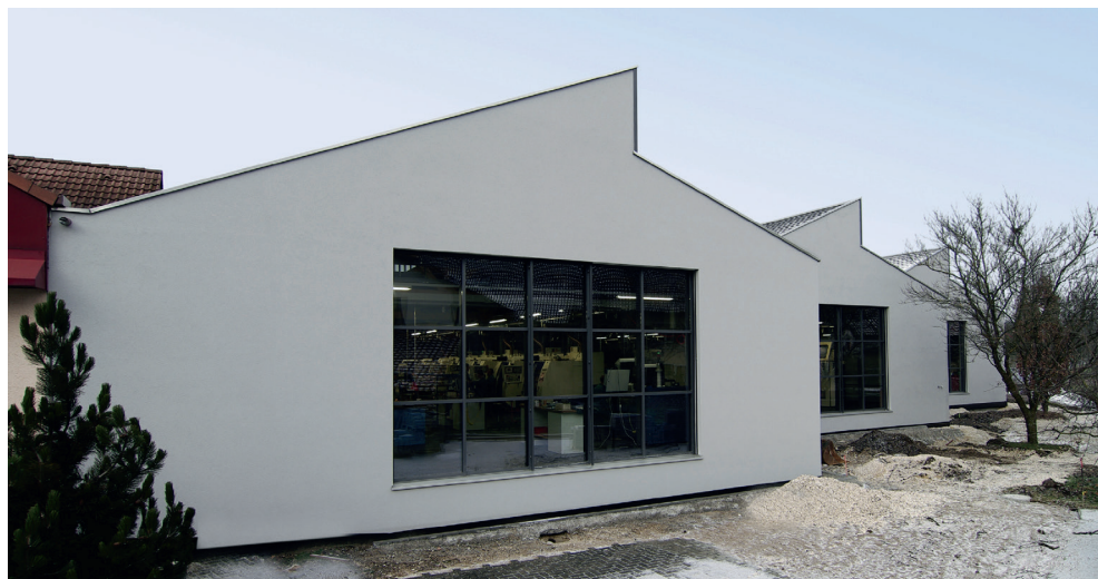
FACADE SUD ATELIERS
